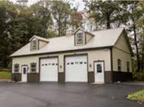
Clay roof, Bronze trim & wainscoting, & Light Stone sides
